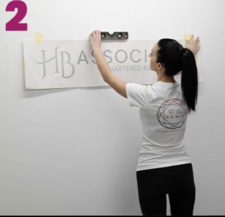
2 USE SPIRIT LEVEL TO ALIGN VINYL
